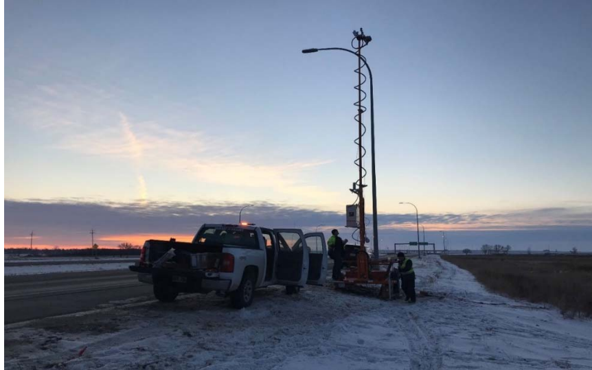
Initial deployment of a portable road-weather and traffic information system in Manitoba
